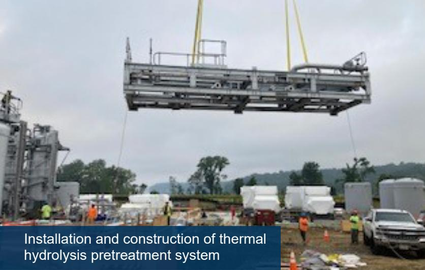
Installation and construction of thermal hydrolysis pretreatment system
