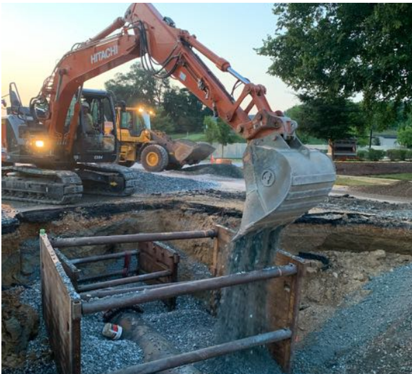
Emergency repair of a 30-inch water main in Prince George’s County
