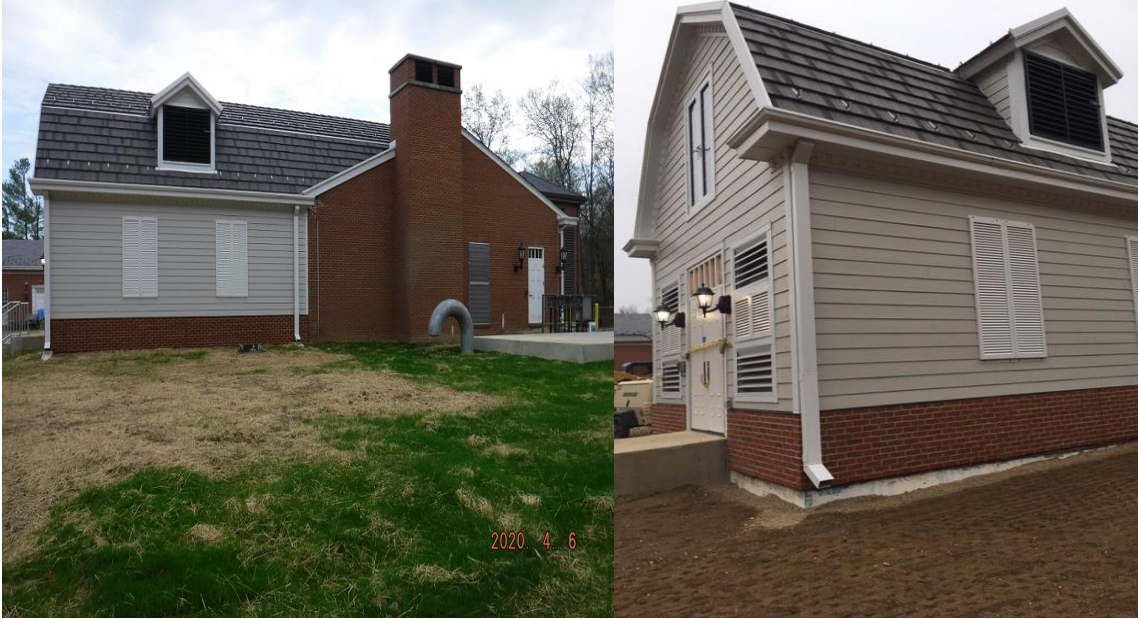
New Electrical Room with 6 Variable Frequency Drives (VFD) and Process Control Equipment
