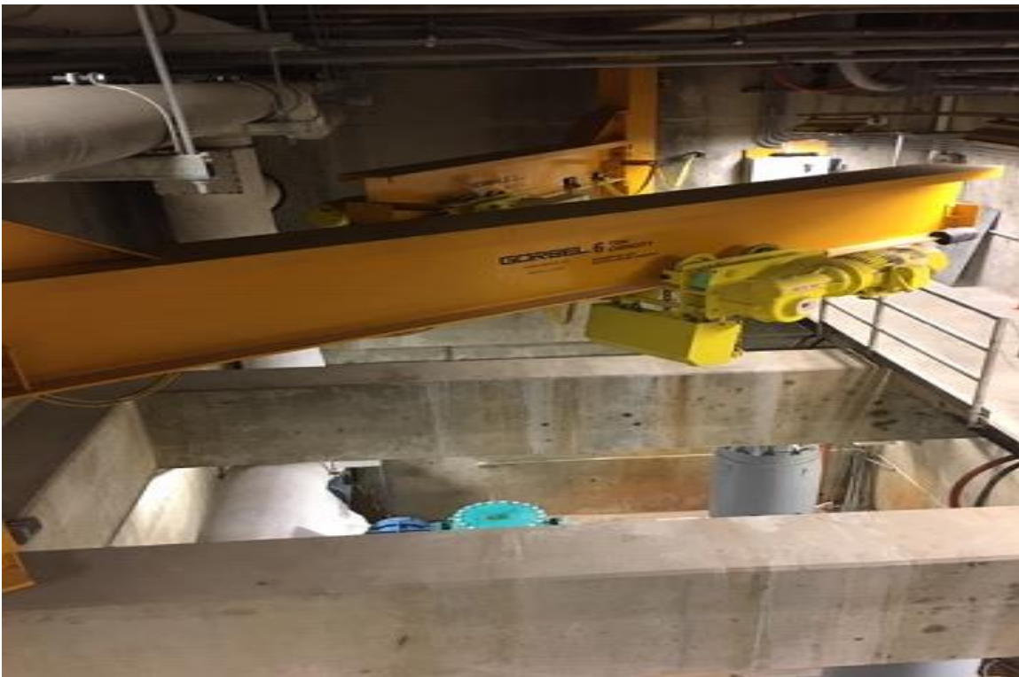
New cranes to remove pumps
