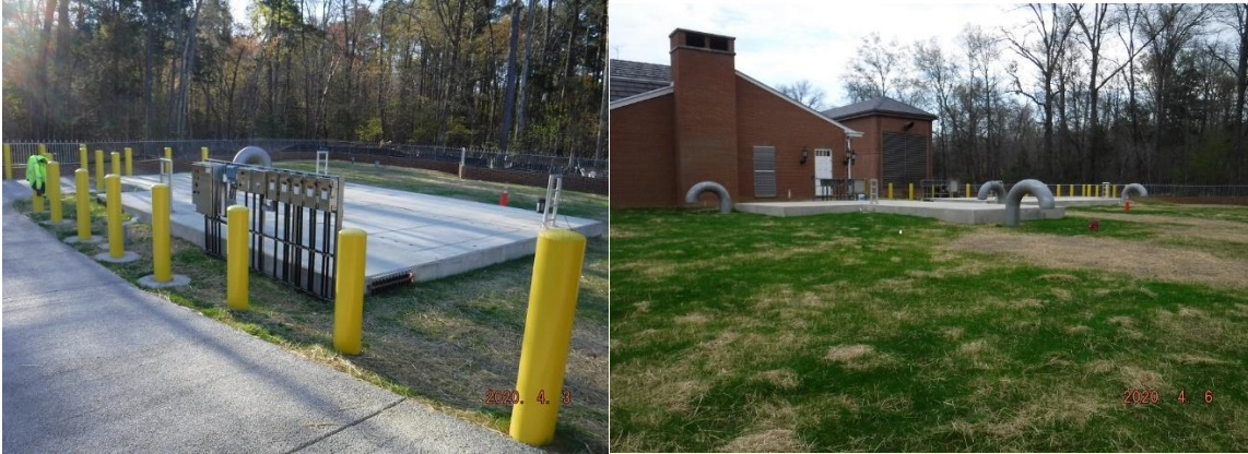
New West and East Valve Vaults
